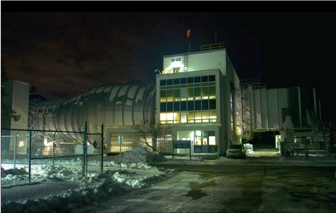
Photo 2.1: Outside View of the NRC Wind Tunnel Facility
