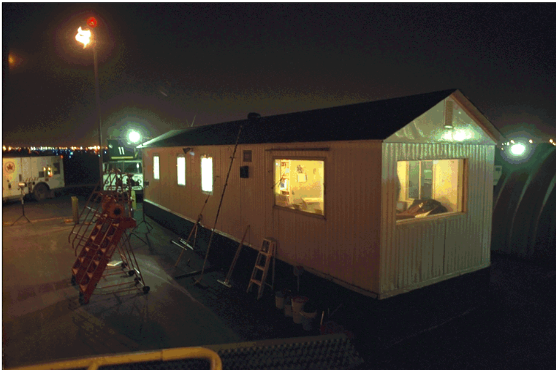
Photo 2.6: Air Canada Deicing Control Centre at East Pad
