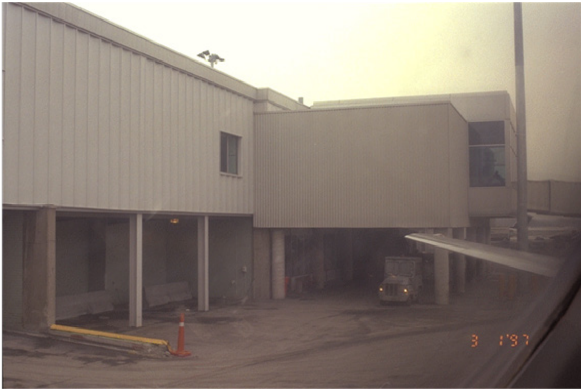
Photo 5.15: View of Wing from Flight Deck - Closed Window (B737-2)
