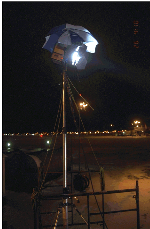
Photo 2.12: Mast Lighting Used for Aircraft Illumination
